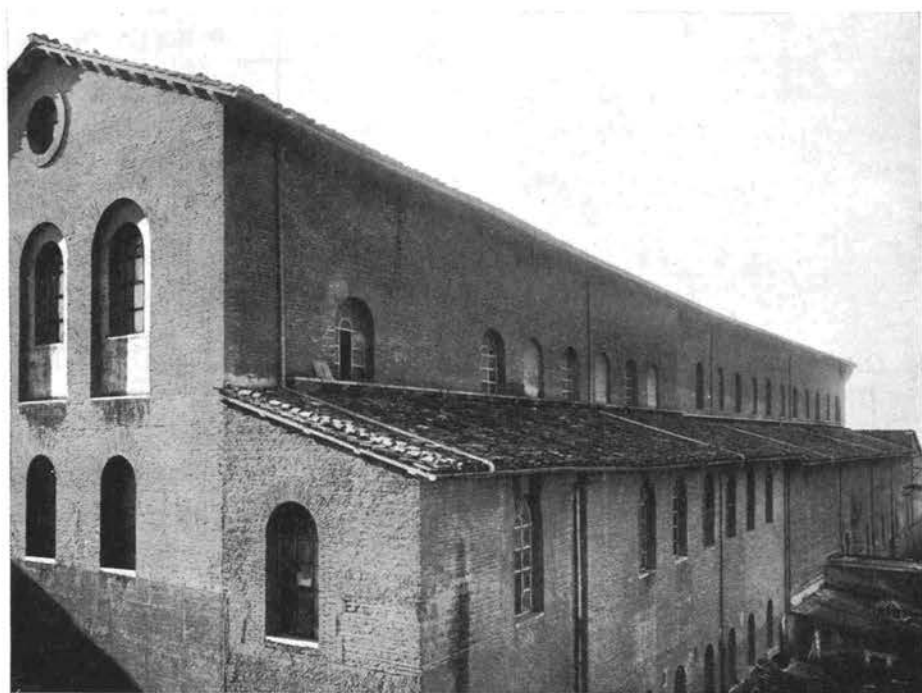
Fig. 29 — S. Lorenzo f.l.m. East basilica, east facade, south flank, and south clerestory from southeast, 1934 (Photo: Sansaini).
